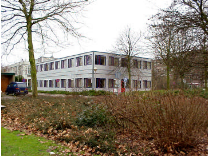
Fig.1: A temporary office section was added to AMOLF in 2001.
